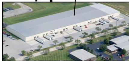
300 Industrial Drive 126,500 SF AIB Certified Food Grade
